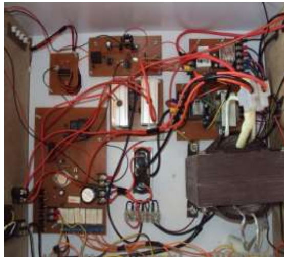
Figure 17: Picture of the Implemented UPS
