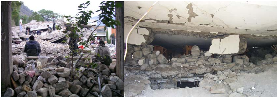
Figure 1. Pakistan earthquake 2005, locals attempting to search for survivors in a collapsed girl's college. The structure was in unstable condition; excavation and lifting machineries were prohibited from the site. (Pictures taken on site by author during mission)
