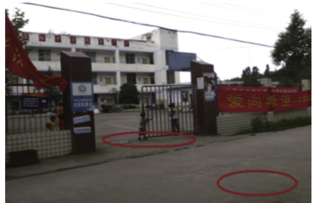
Figure 5. Children are playing around the old damaged school building and traffic roads.
