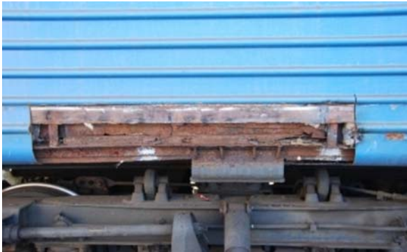
Fig. 4. Deformation of side sill at 2500 mm length of non-boiler side, bend 20 mm
