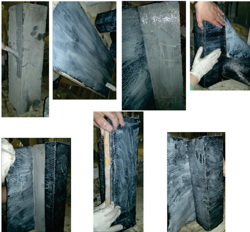
Photo 1: Procedure of wrapping with CFRP
