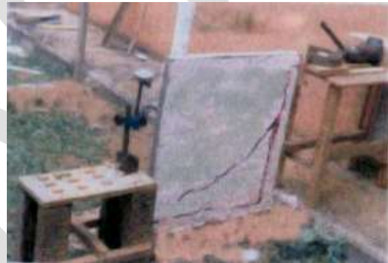
Figure 3: Failure Mode of MF1 Frame
