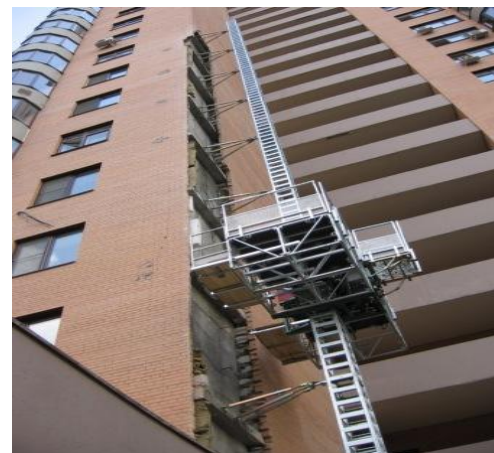
Picture 1 - Demonstration of problems with multi-layer brick facades. [6]
