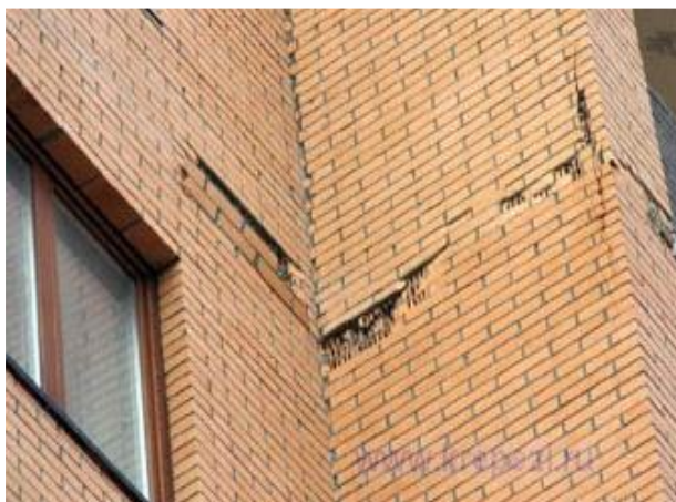
Picture 1 - Demonstration of problems with multi-layer brick facades. [6]
