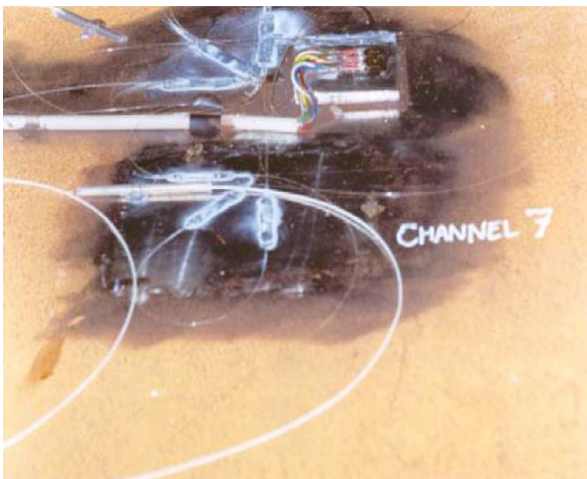
Fig. 2. Installed optical fibre sensors on steel structure.
