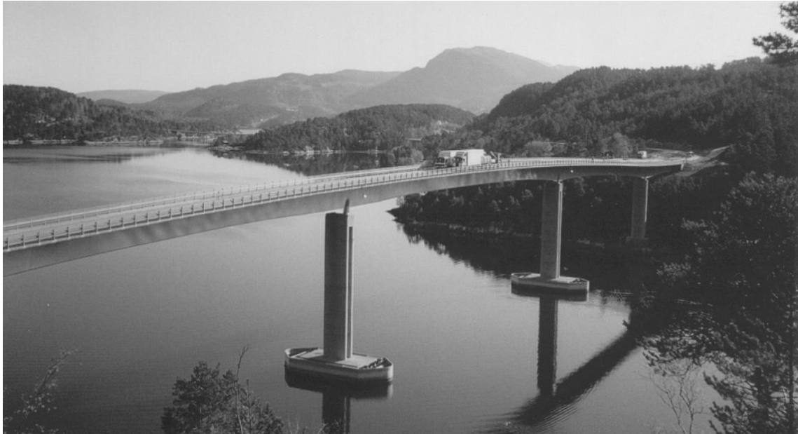
Fig. 12. Mjosundet Bridge used for the field trials.
