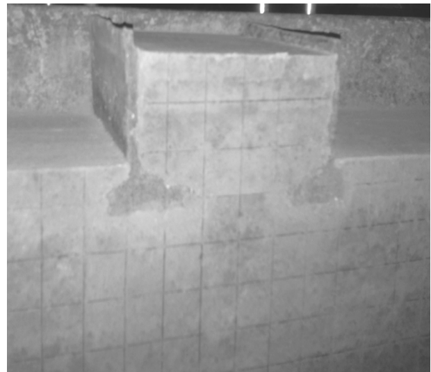
Fig. 12. Strain of the retaining wall model with piles after load application
