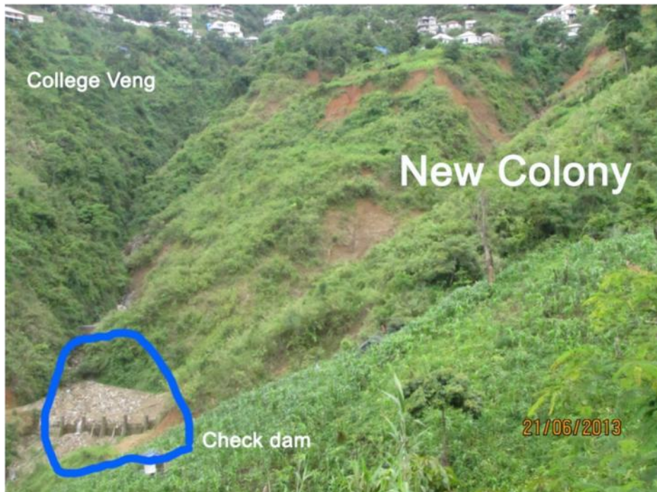
Photo plate 4. Check dam at the toe of College Veng - New Colony area, constructed by DRDA, Saiha.
