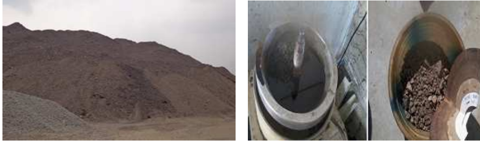
Figure 2: Stock Piled Milled RAP Materials Figure 3: Extraction of Bituminous Mix
