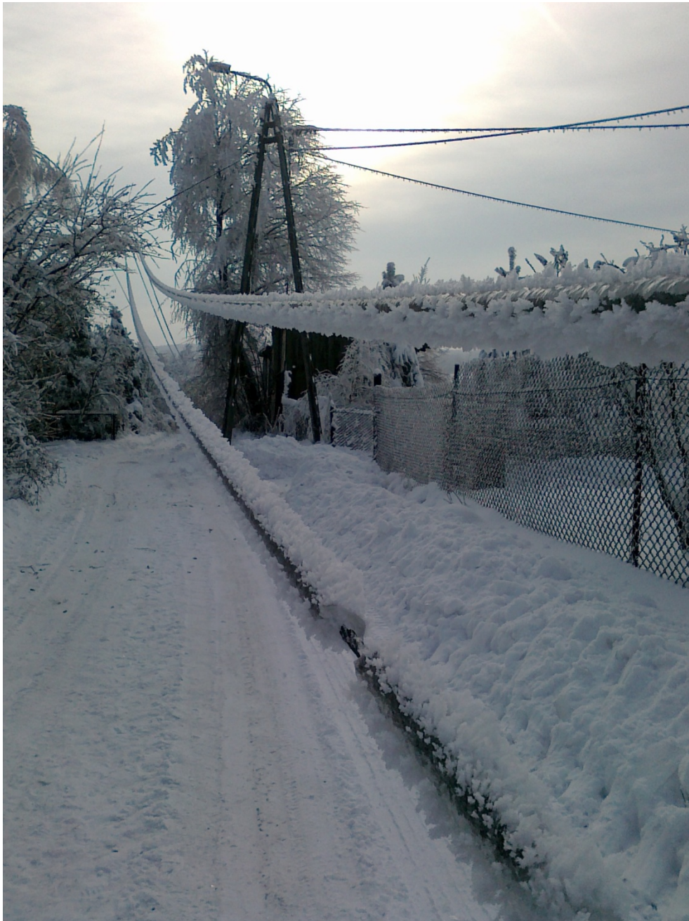
Figure 4. The effects of icing In Janow Community Source: Archive of Janow
