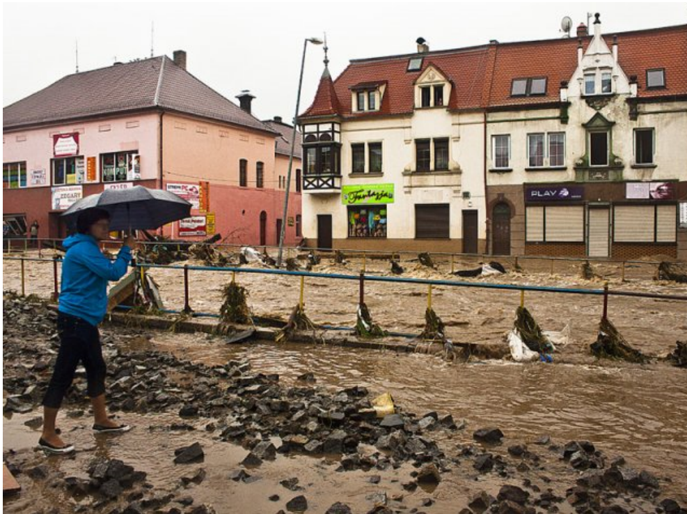
Figure 3. The street after the flood in Bogatynia city
