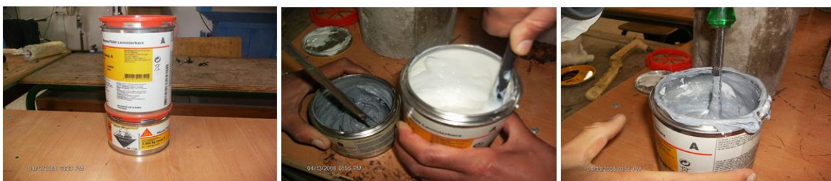
Fig 2. Preparation of resin (SIKADUR 330).
