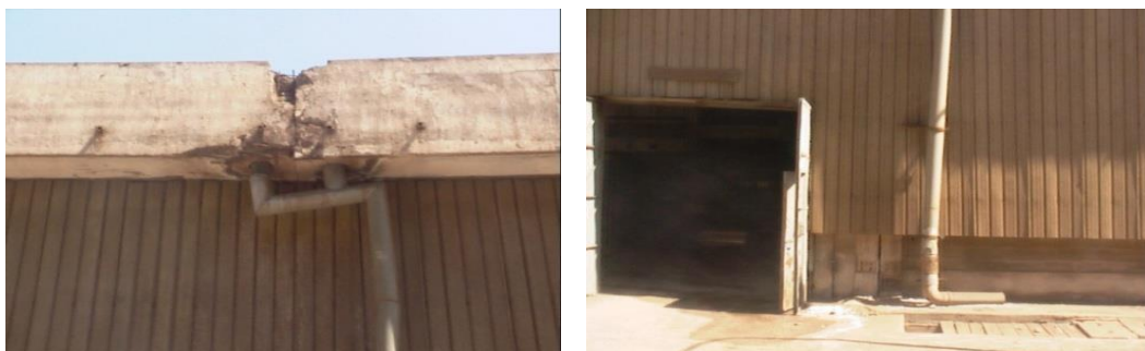
Fig. 8 –Seismic joint seen from the outside at the top and bottom
