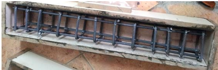
Figure 2 Steel reinforcement cages and the mold
