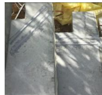
(f) fulling grooves with epoxy
