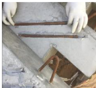
(e) Installing the steel bars
