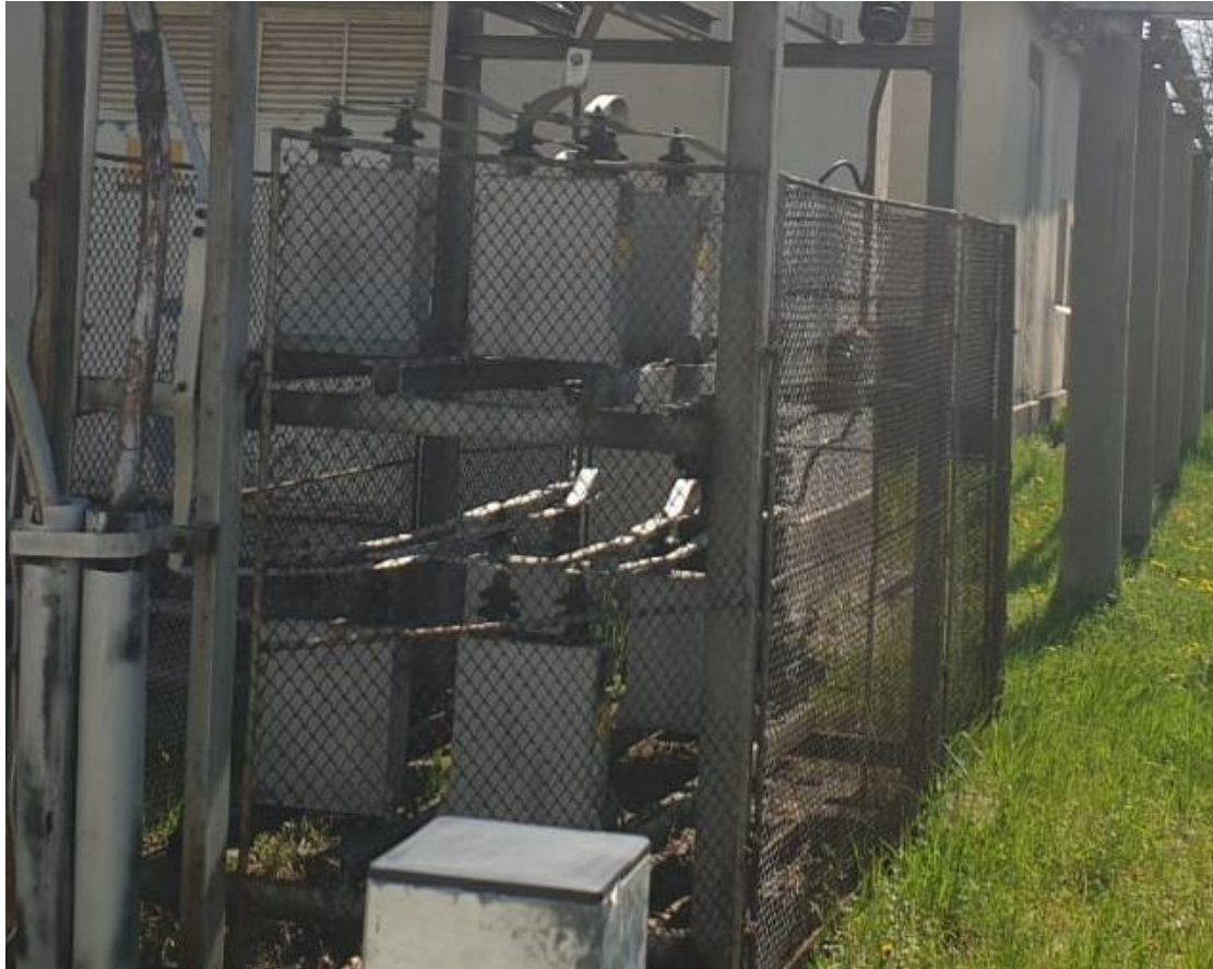
Fig. 2. PCBs capacitors in Maramureş county
