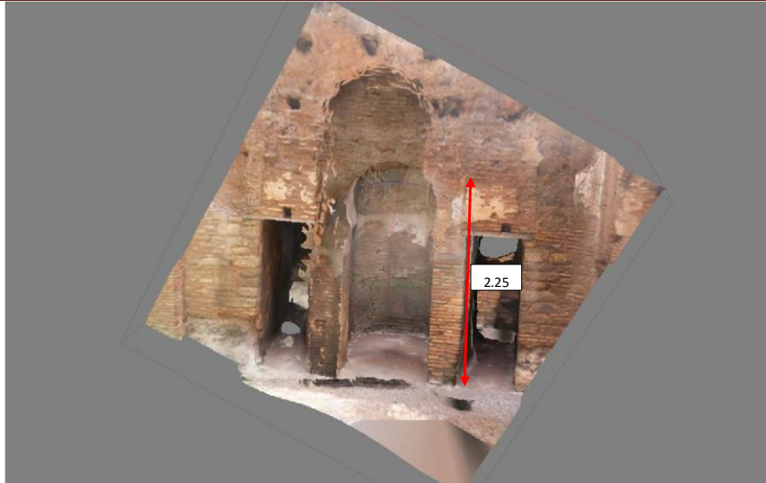
Figure 7. Point cloud as a support for measuring (source: Authors).
