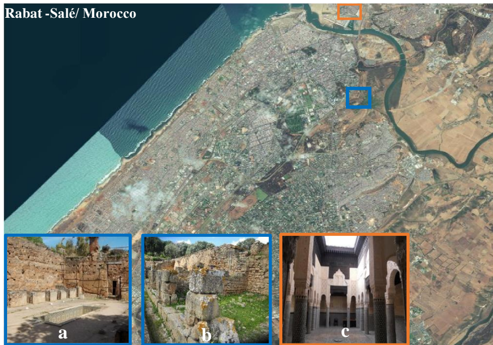
Figure 1. Study area, a) Madrasa of Abu-Al-Hassan, b) The Roman site, c) AlMadrasa Al-Marinia. (Source: Google earth pro).
