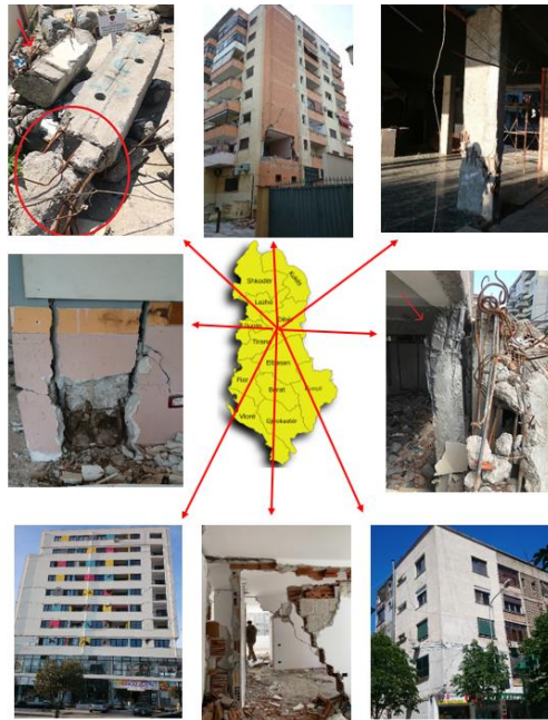
Fig. 2 Consequences to reinforced concrete buildings during the 2019 Albania earthquakes
