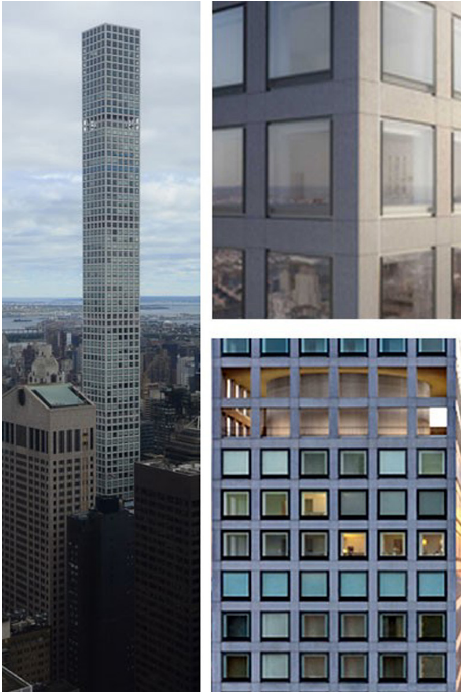
Fig. 12. 432 Park Avenue (photograph by authors)
