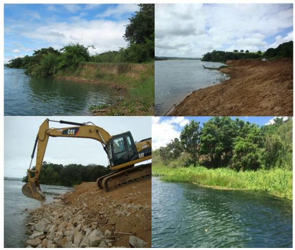
Figure 10. Lower São Francisco Riverbank recovery, Northeastern Brazil, through soil bioengineering technique called Vegetated riprap, from 2010 to 2018.
