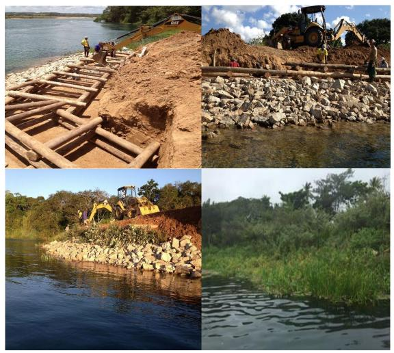
Figure 11. Lower São Francisco Riverbank recovery, Northeastern Brazil, through soil bioengineering techniques called Crib-wall, from 2013 to 2018.
