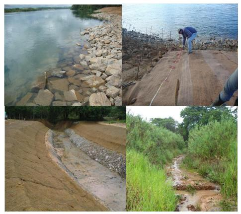
**Figure 8.** Use of geotextiles, with riprap and gabion as toe protection, on the banks of the São Francisco and Paramopama Rivers.
