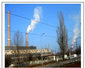
Fig. 21. Overview of the new thermal source operating in the western part of Oradea City from the winter 2016/2017 (new gas turbine installation together with the 25 MWe group upgraded on gaseous fuel).
