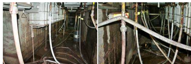
Figure 4. Intervention for increasing flow in girders
