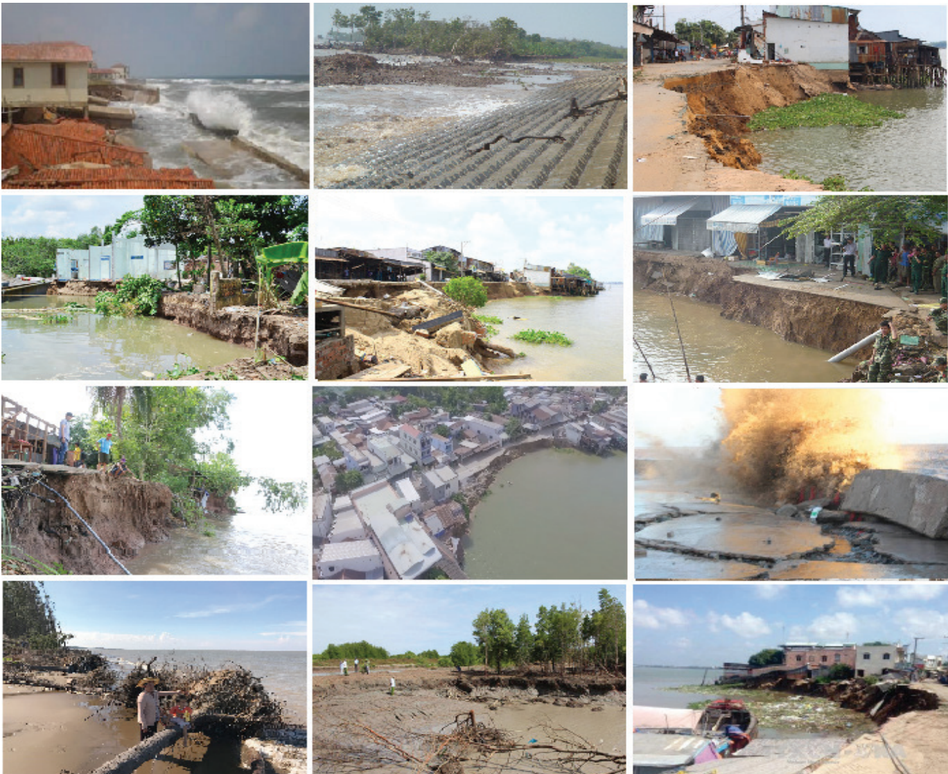
Fig. 9. Some pictures of erosion at river banks and coasts in the Mekong delta (Source: individual information, e-newspapers, and the Internet).
