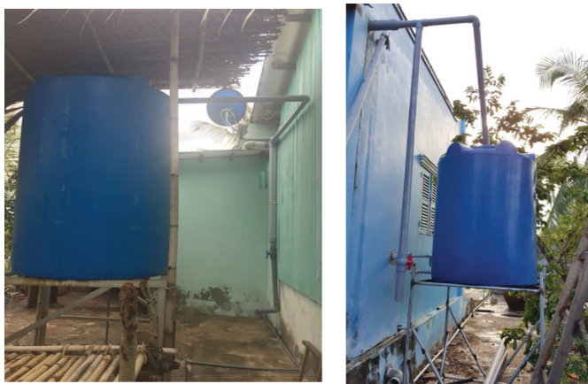
Fig. 3. The 2 pilot rainwater harvesting system in Hoa Dong commune, Vinh Chau town.
