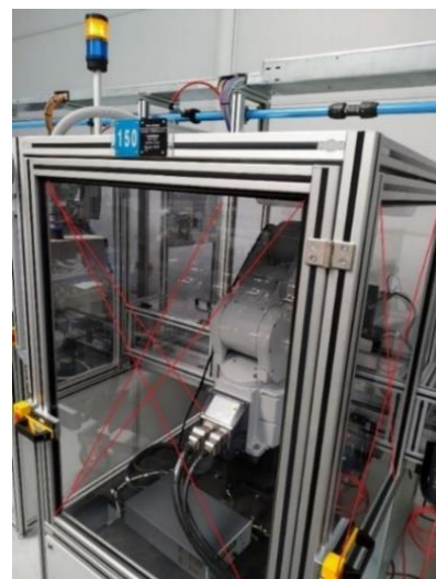
Fig. 2. Fencing of a robotic workplace
