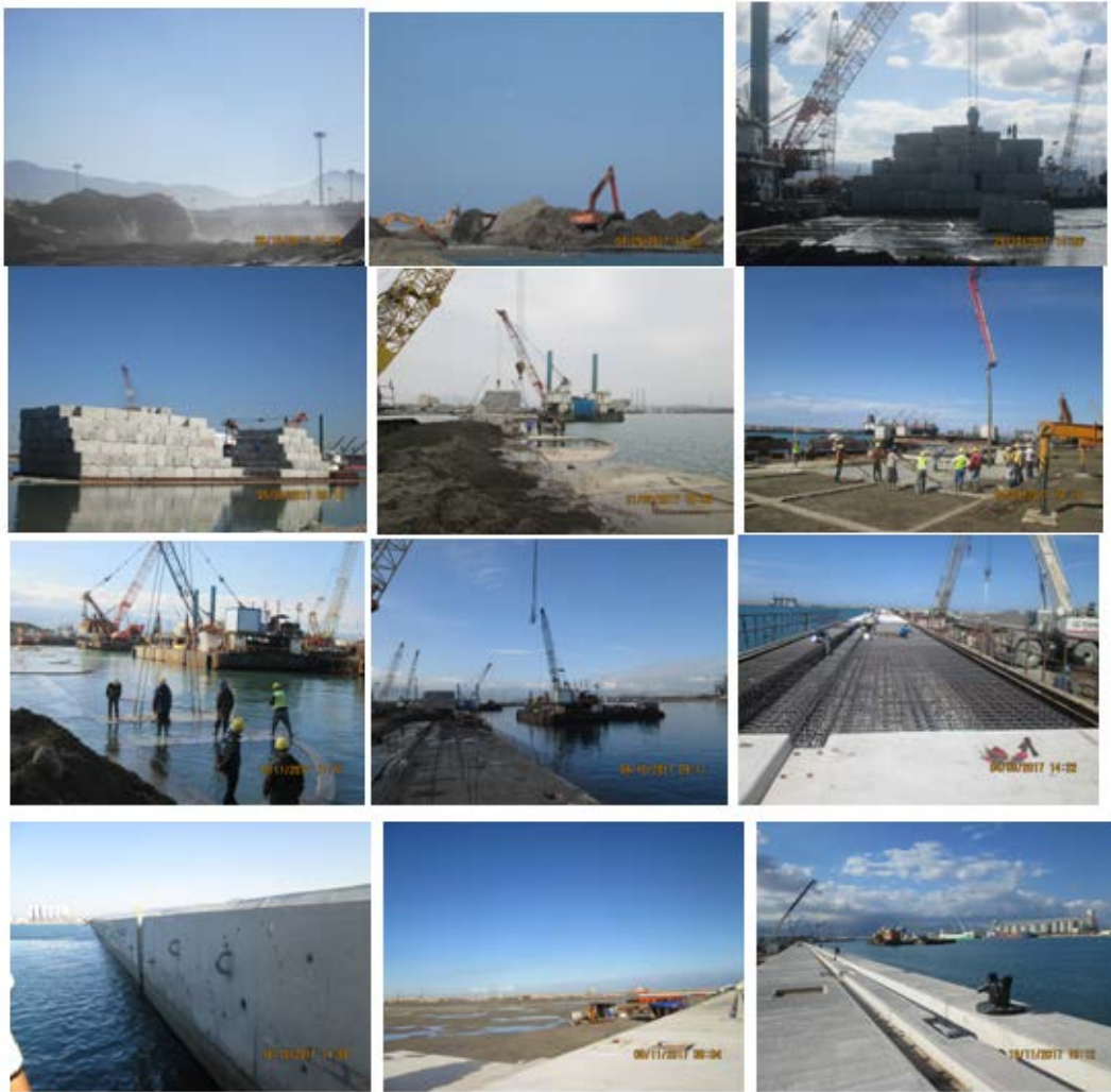
Fig. 18– Photos of the quay wall
