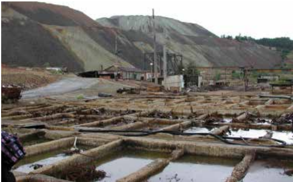
Fig. 2 - 3. A general view of the operation for copper dump bioleaching at Vlaikov Vrah mine
