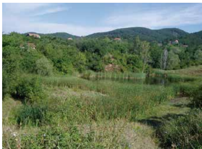
Fig. 9. Treatment of acid mine drainage by constructed wetland in the uranium deposit Kurilo
