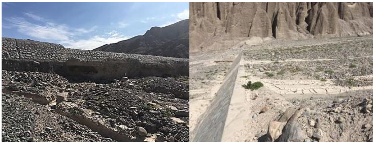
Figure 14. Left: View from downstream of Dike 2, showing the erosion and regressive erosion below the foundation of the dike and its dissipating pool after the debris flow event of 2019. Right: The dike vessel is shown sedimented with solids by effect of the debris flow of 2019.
