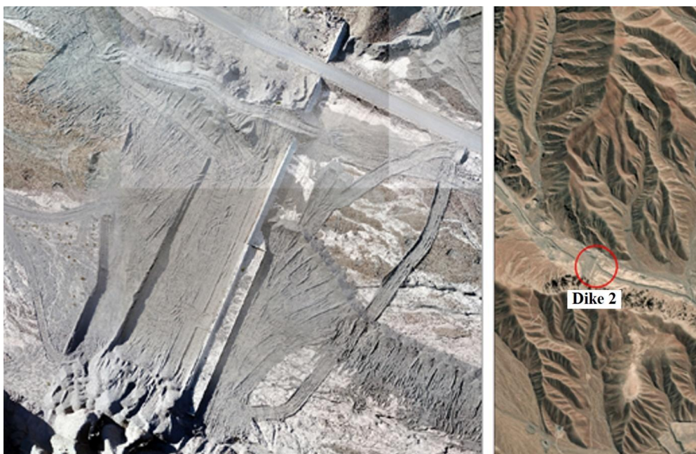
Figure 13. View of drone photogrammetry (July, 2018) of sediment retention dam (Dike 2), located in Mirave's main stream; and operational state of dike and sinkhole before the debris flow of 2019.
