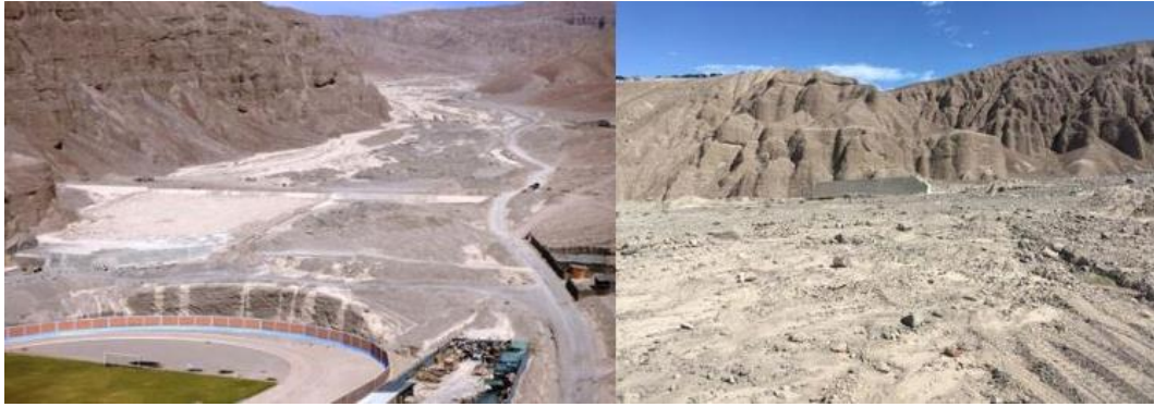
Figure 16. Left: View from downstream of Dike 3 before the debris flow of 2019, where the dike and its dissipation pool can be observed, and immediately downstream of the location of an additional protection containment wall, and football stadium. Right: The debris flow of 2019 devastated and overwhelmed the structure of Dike 3 and the football stadium, partially collapsing the retaining wall.
