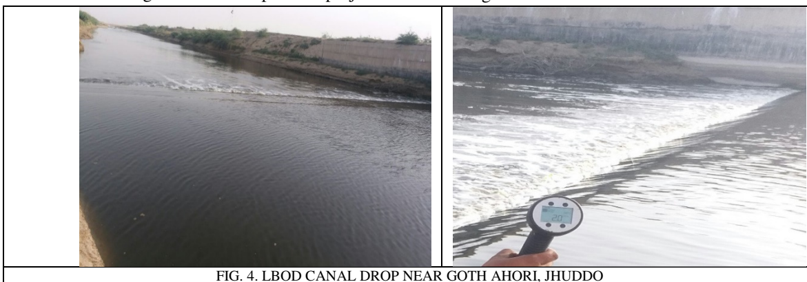
FIG. 4. LBOD CANAL DROP NEAR GOTH AHORI, JHUDDO
