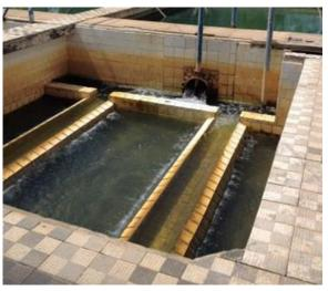
**Figure 1.** Image of one of the filters during the backwash process. **Source:** Samae (2016).
