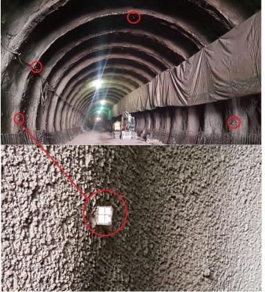
Figure 6. Tunnel deformation target.
