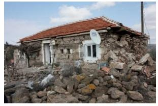
Figure 11b: Example of damaged beam-less structure
