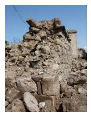
Figure 4: A Section from Bearing Stone Walls Constructed in the Region
