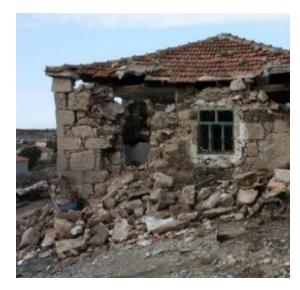
Figure 17: The damage caused on the wall by the chimney
