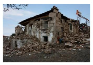
Figure 9: Damage to a Structure with Low Strength Soil Mortar
