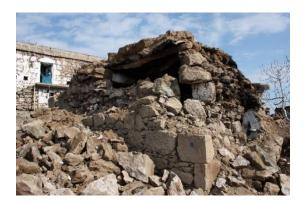
Figure 8b: Example of a Damaged Wall with Double Wall in a Structure in Yukarıköy
