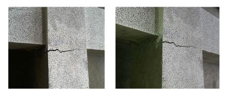
Figure 11. Cracking under concrete beams. Source: [1]
