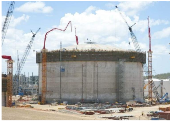
Figure 5: Visualization of an LNG tank construction [67].
