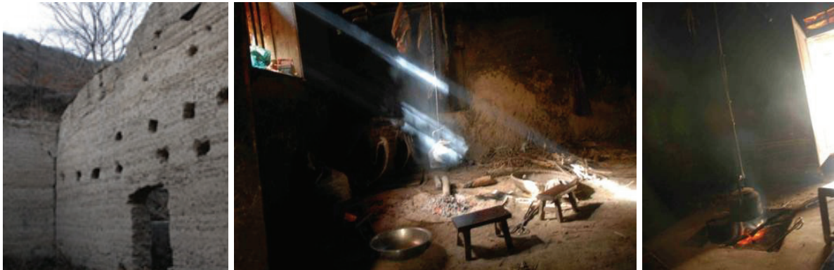
Figure 2. An abandoned farmhouse
