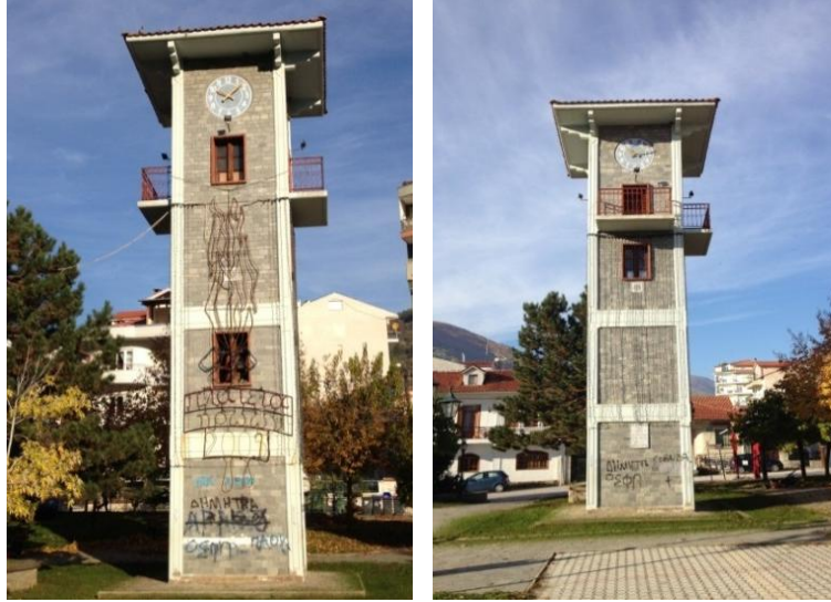
Fig. 1. Surfaces of the building
