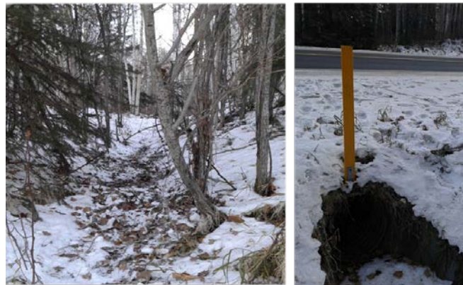
Figure 3. Prominent water track intercepting with the Goldstream Road. Water flow in the track has eroded the finer sediments over time so that the track resembles a rill.
