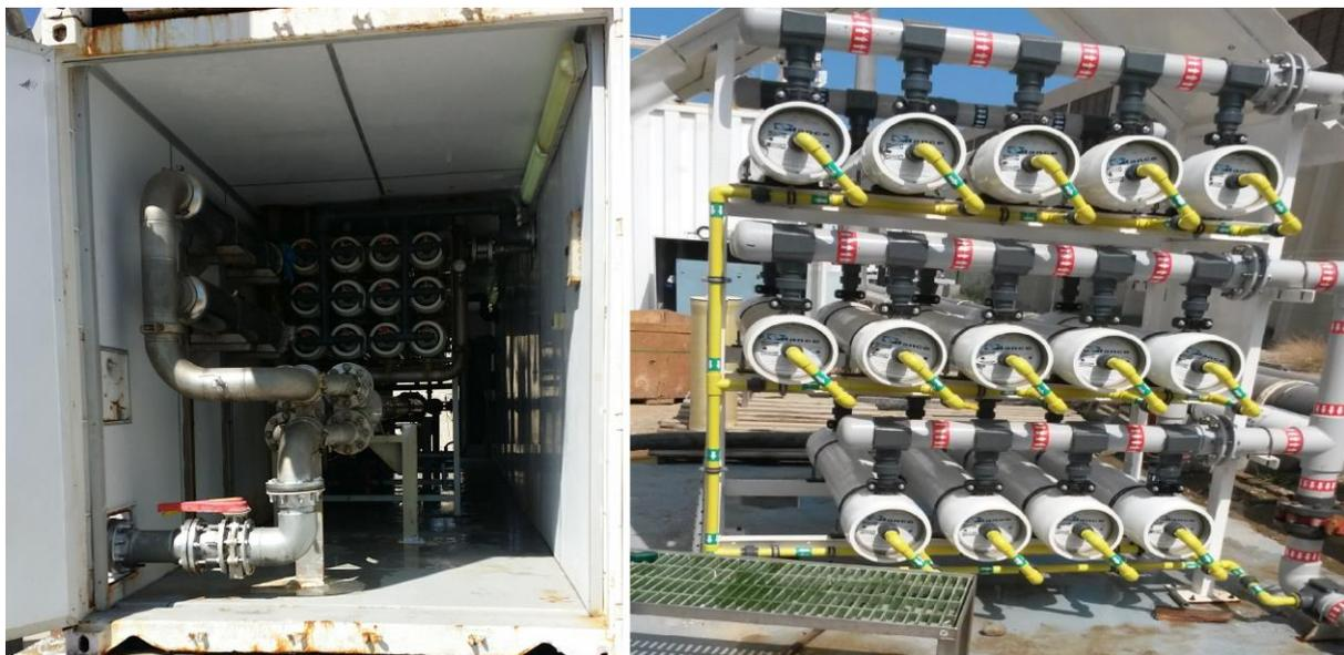
**Figure 3:** RO desalination plant in a mobile system (photo: Bashitialshaaer, 2015)
