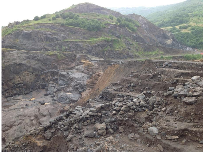
Figure 4: Partially Collapsed Dam at Samsun Flood, 2012.
