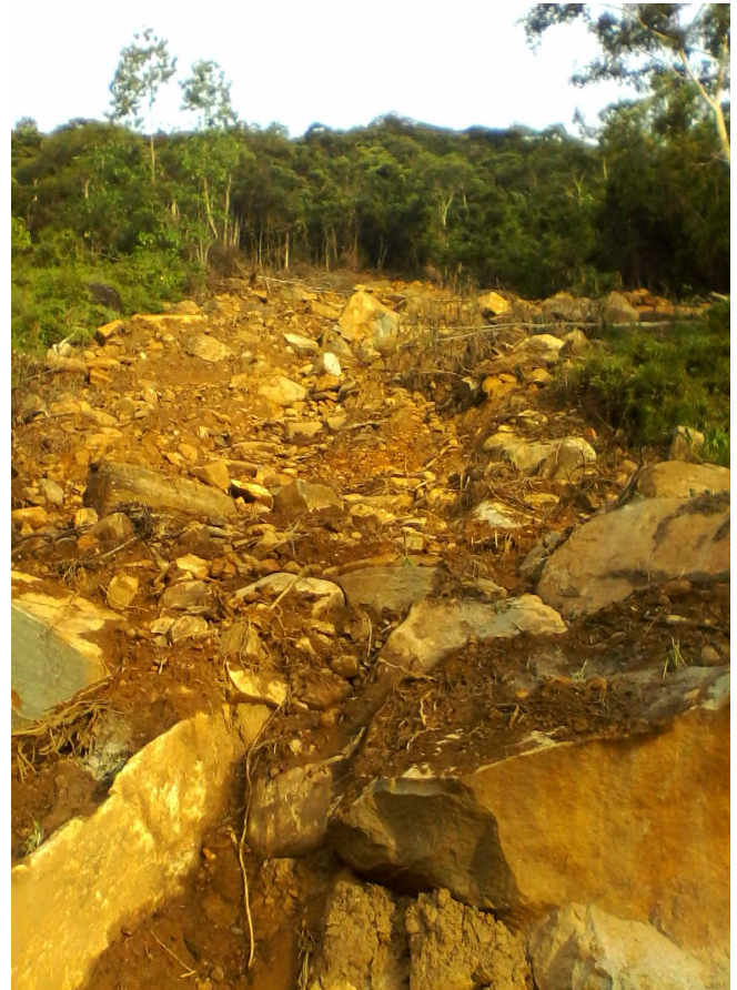
Fig. 9. Landslide due to heavy rainfall.
