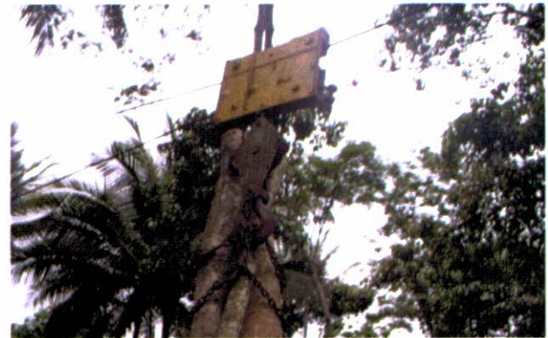
Gambar3. Angkut muatan Figure 3. Load transportation
