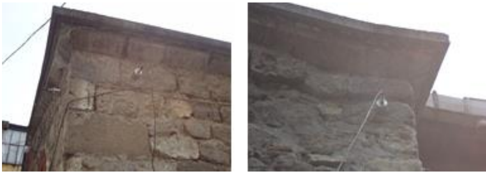
Fig. 8. The images of measurements of Molla Siyah Mosque before the restoration
