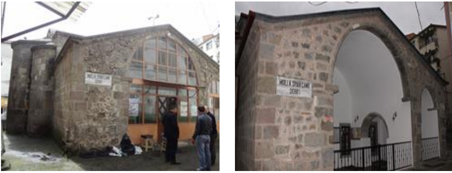
Fig. 2. Images of Trabzon MollaSiyah Mosque before and after the restoration
