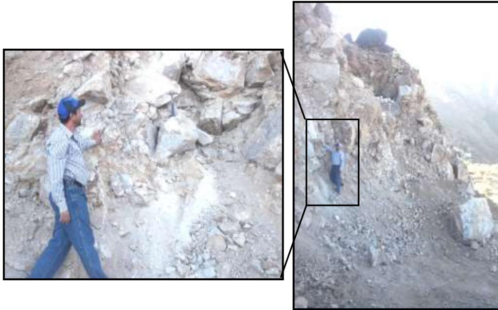
Fig. 5 Weathered granite slope at location No. 20
