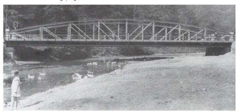
Figure 6 The first welded bridge mounted across the Bârzava River at Stavila
