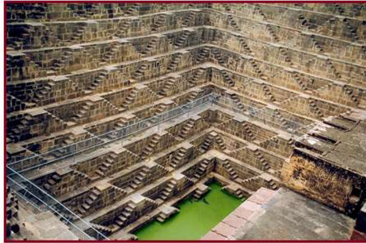
Fig.2. Step wells in India
