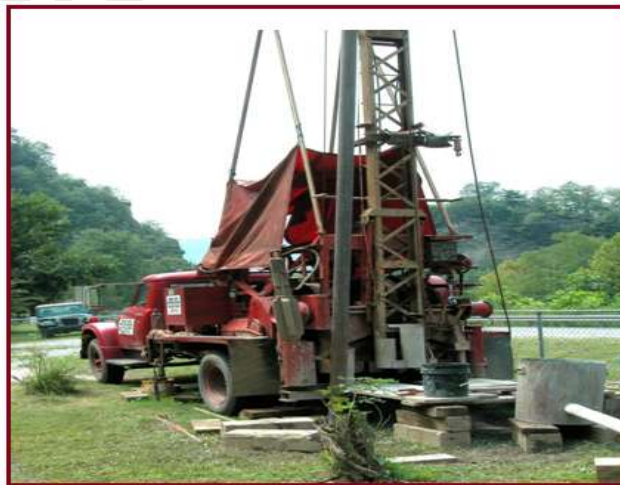
Fig.8. Rotary drilling technology in 20 th century.
