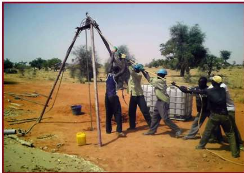
Fig.5. People use drilling spring poles for water Harvesting.
