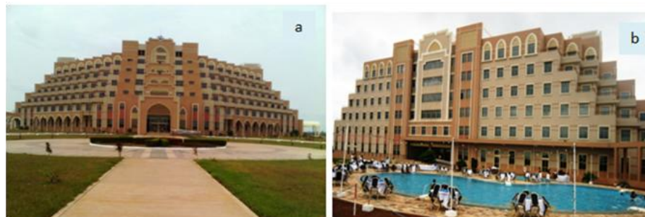
Figure 2. Picture of the Hotel of the Parlementaires (HDP); a) front side; b) back side
