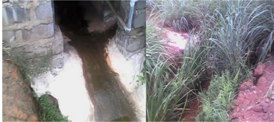
Figure 4. Discharge of paint leftover from the Hotel onto the soil
