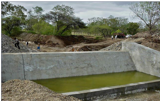
Figure 7 Cement Nala Bund
