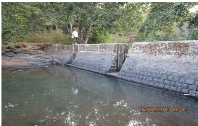
Figure 8 Stone Masonry Bund
