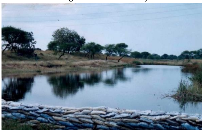
Figure 10 Vanarai sand soil/bag Bund
