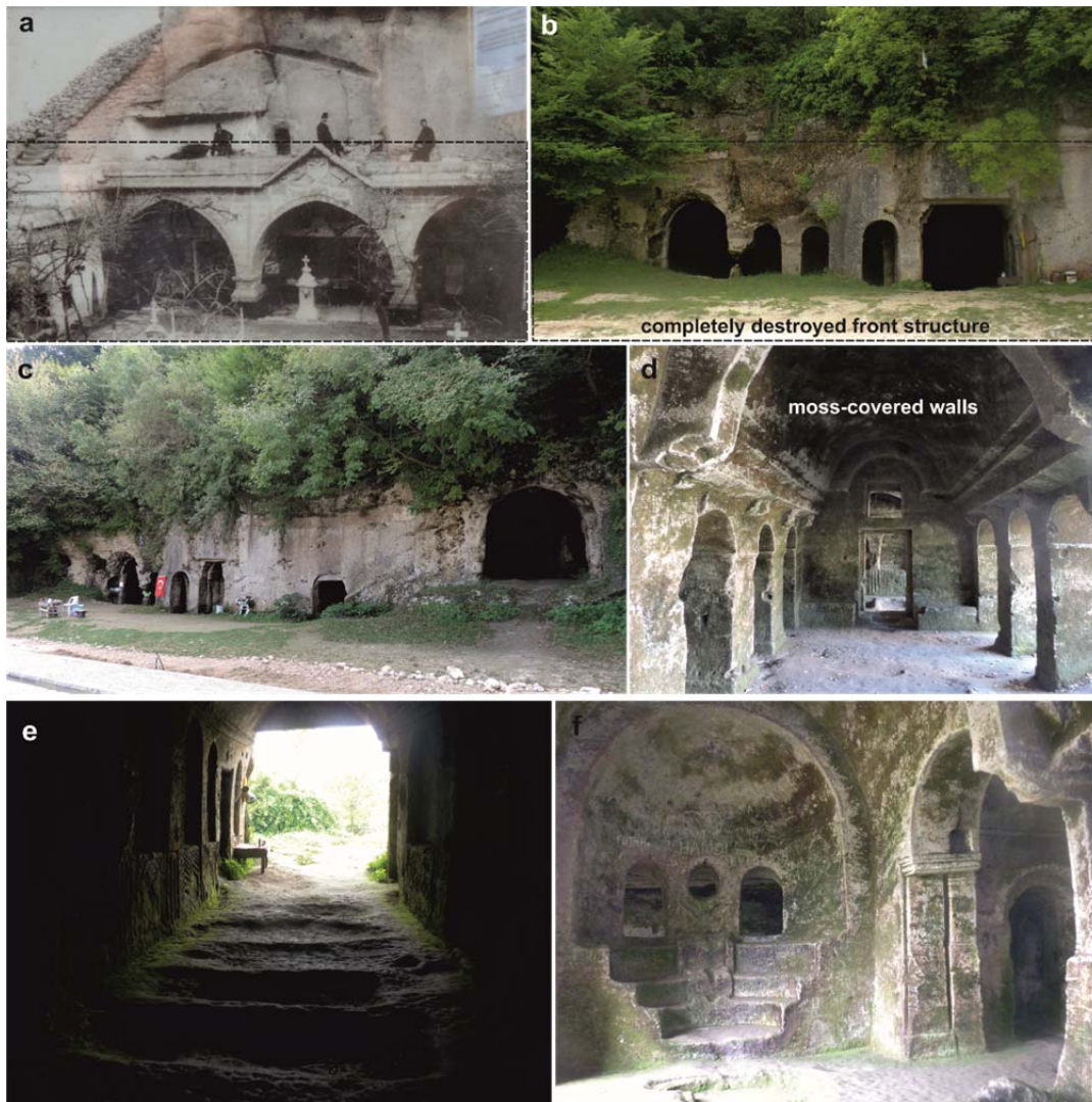
Fig. 2. Views of Aya Nicholas Monastery. (a) Front of the rock-cut monastery during pre-Republican period, (b,c) intense destruction and biologically-induced deterioration in front of the heavily-destroyed monastery walls, (d) moss-covered walls, (e) ruins of tombs, and (f) abscissa section near entrance to the monastery.
