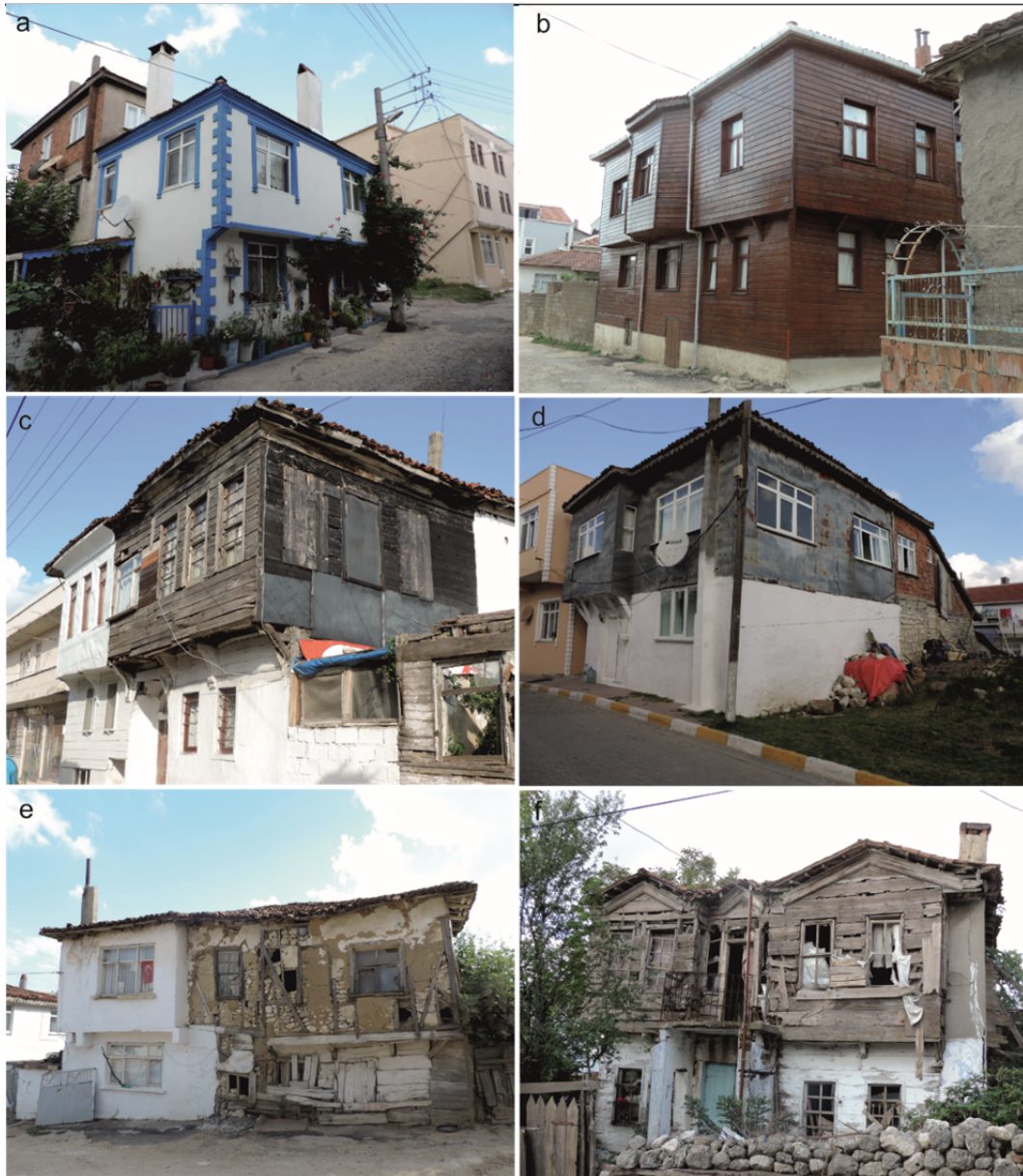
Fig. 4. Views of Kıyıköy Houses used for residential purposes at present and those that have been largely destroyed. (a,b) completely-restored houses, (c,d), incompatible interventions on the original architectural texture of building facades, and (e,f) completely ruined houses.
