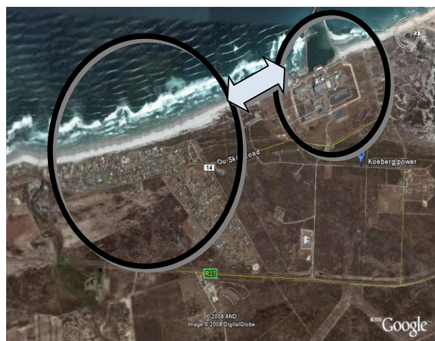
Figure 4: The relationship between Koeberg nuclear power plant buildings and touristic villages viewing the ocean [6].
