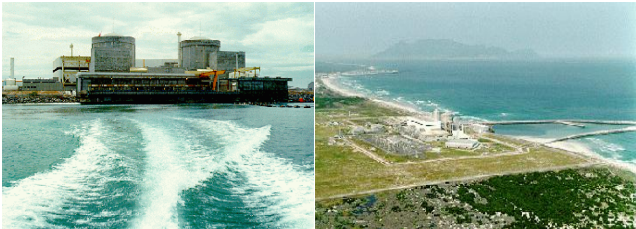
Figure 5: The external formation of the Koeberg nuclear power plant, South Africa [7].
